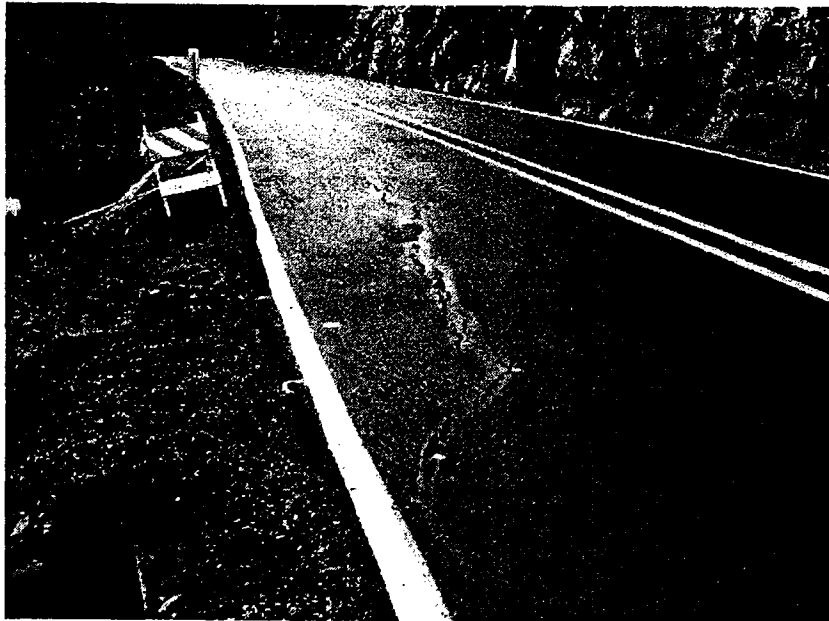
Photograph 6: North side of Sweet Creek Road showing pavement cracks from settlement of embankment.
