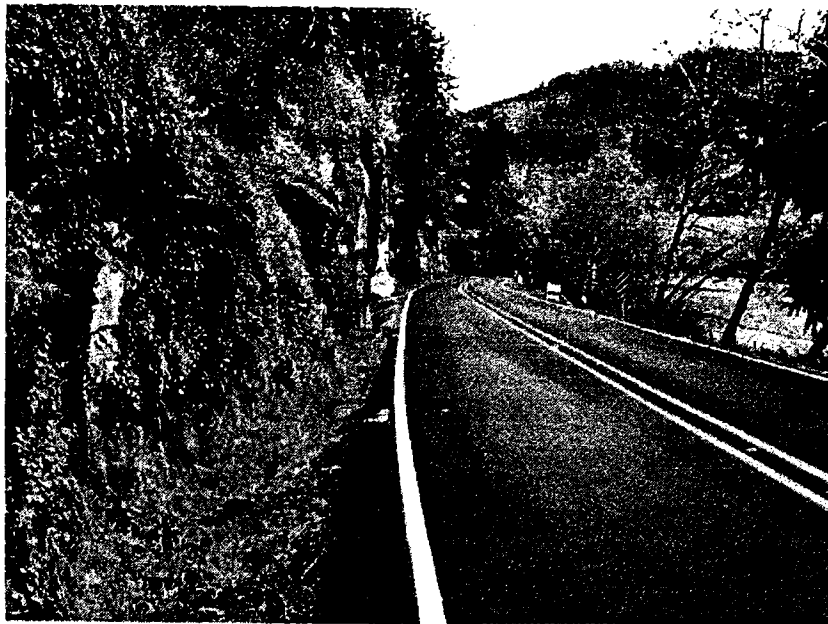
Photograph 10: Looking West along Sweet Creek Road. Steep rock embankments can be seen on the left and the Siuslaw River on the right.
