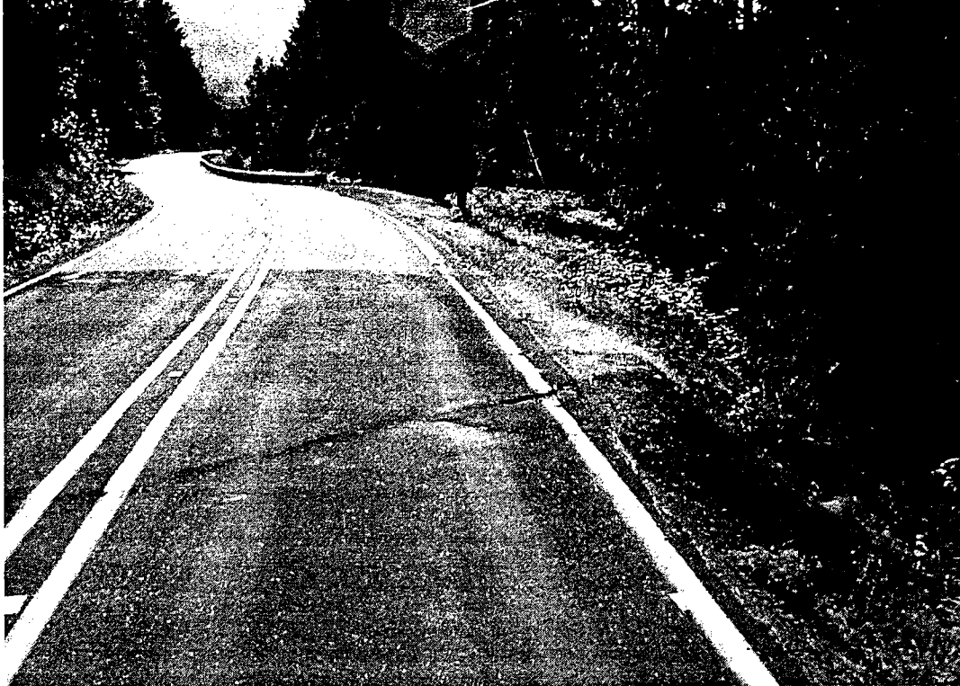
Kitson Springs Road MP 2.7 Looking South
