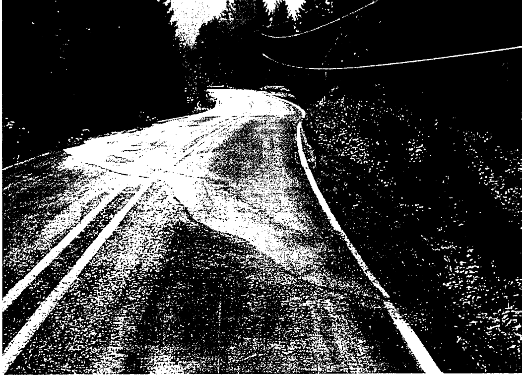
Kitson Springs Road MP 2.65 Looking South
